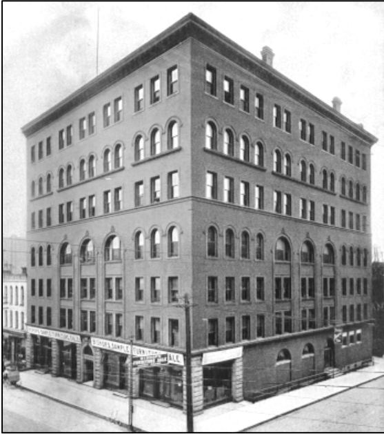
21-23 07/19/62 ---- Capitol Bishop Furniture loading dock.
